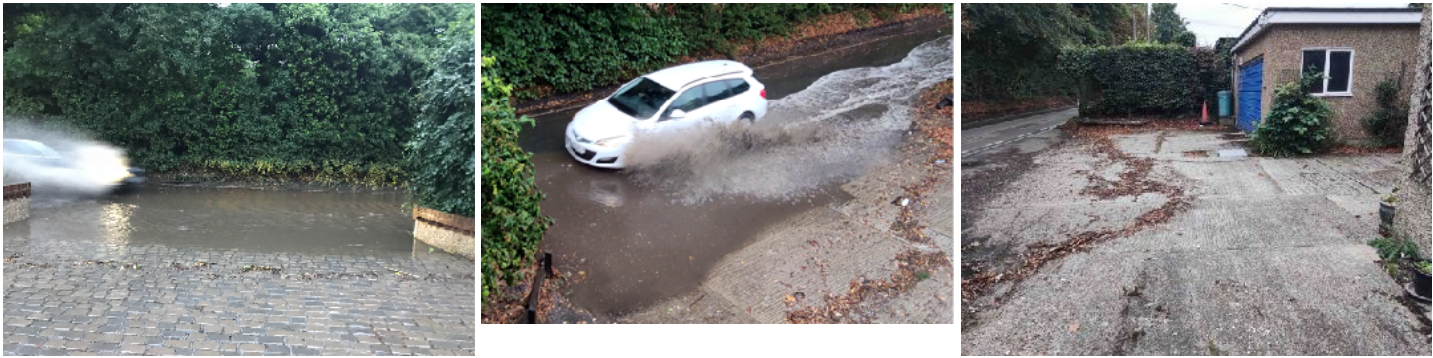
Photos above show surface water flooding of Valley Road in this area (left, June 2019 and centre, August 2022) the “tide mark” of debris following water overspilling the new kerb (right, August 2022)
