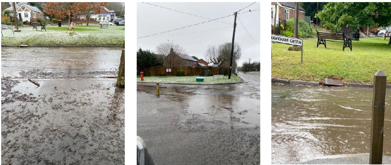
Photographs showing the village green area, (left and centre) January 2021 - with debris showing extent of flood width - and (right) June 2021. These are after the repair work was carried out.
